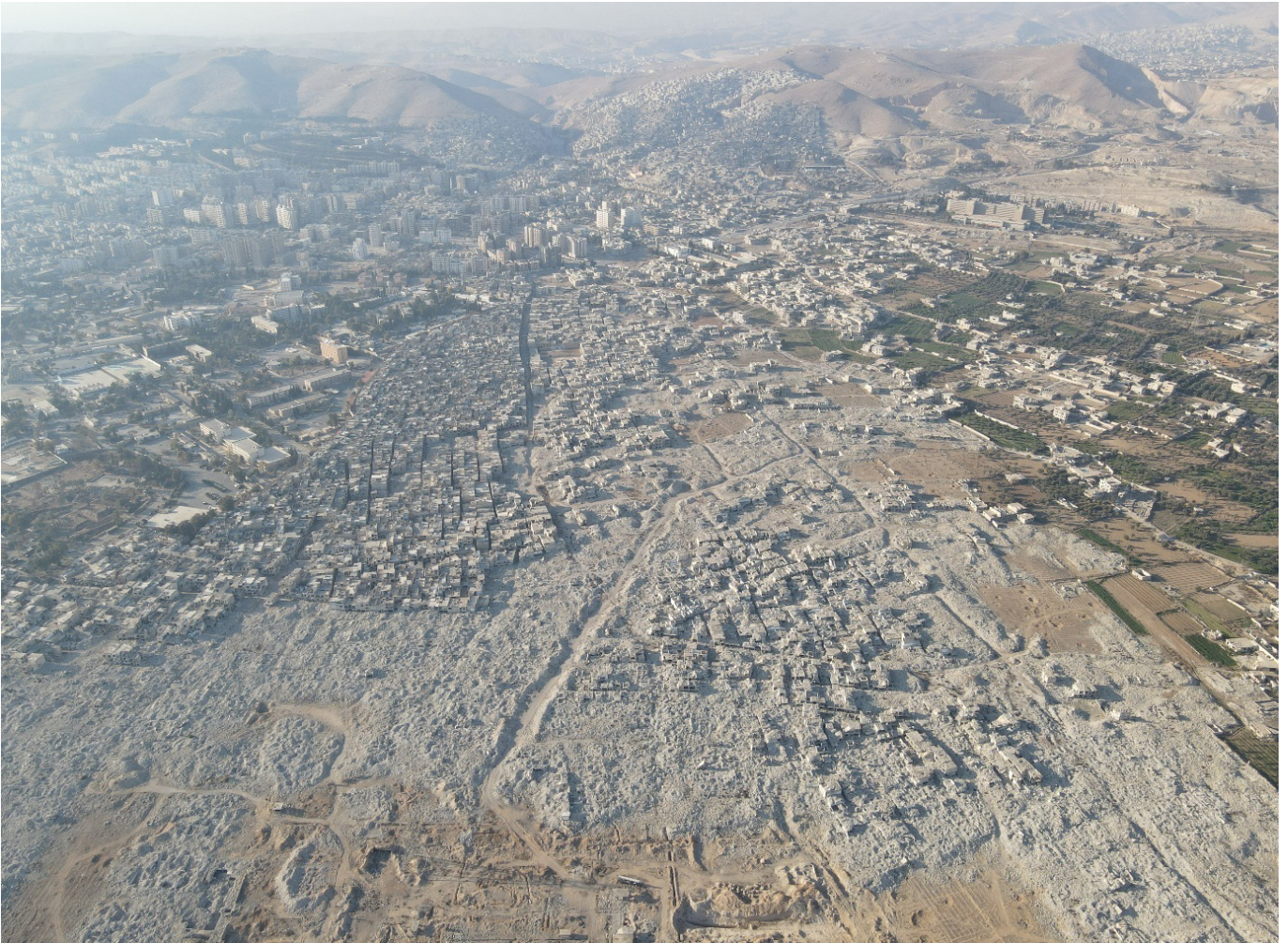
Figure 6 Aerial view of Eastern Damascus, Al-Qaboun. Source: Mulham Team, 2025.
